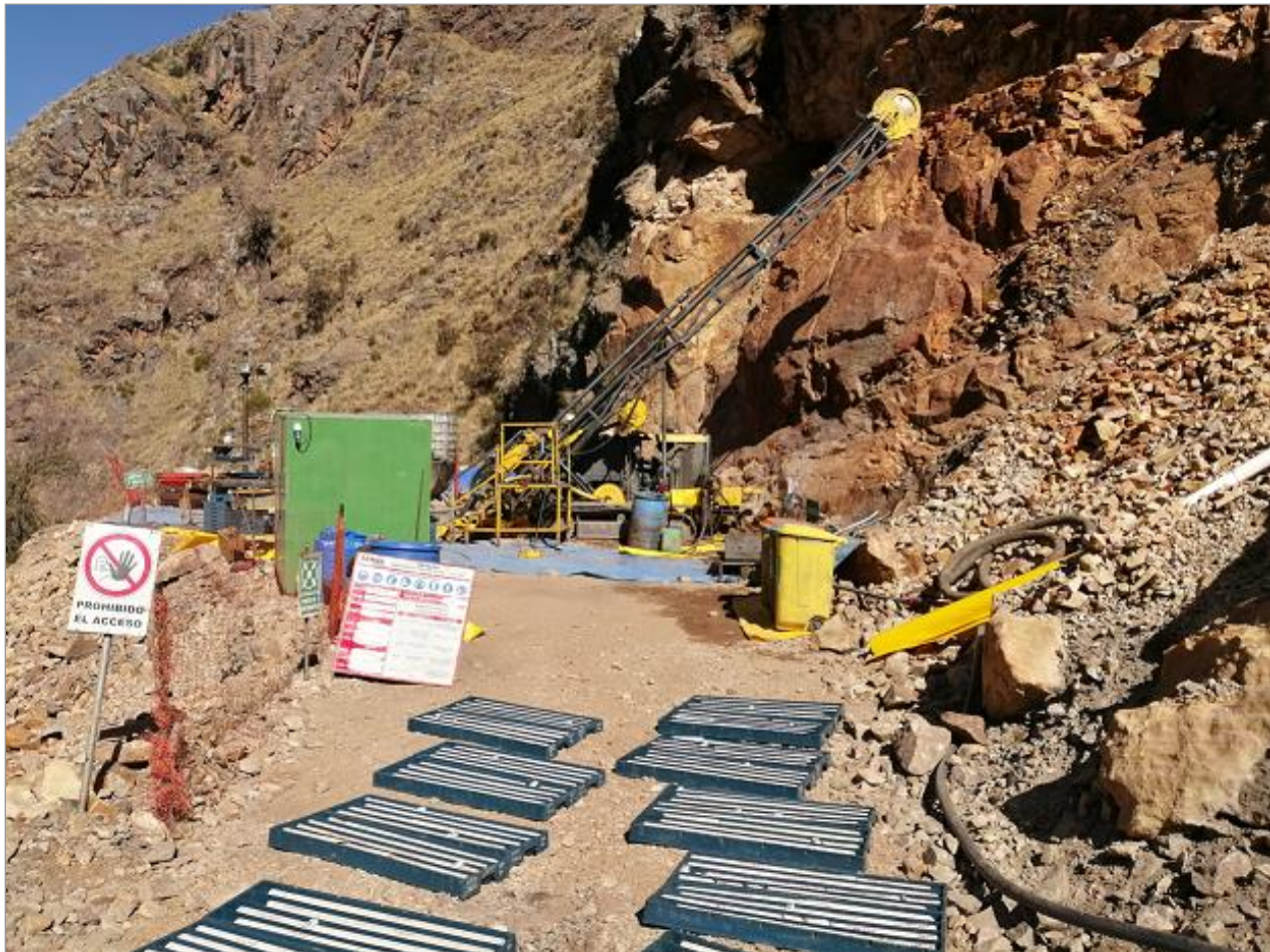
Figure 10.3 Jisas North prospect drilling, showing “quicklog” process
